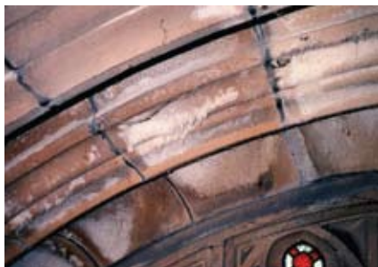
Figure 4 Thin needles of salt extruding from the top of a window arch. A slipped roofing slate punctured the copper roof gutter, allowing rainwater to wash salts into the stonework.
