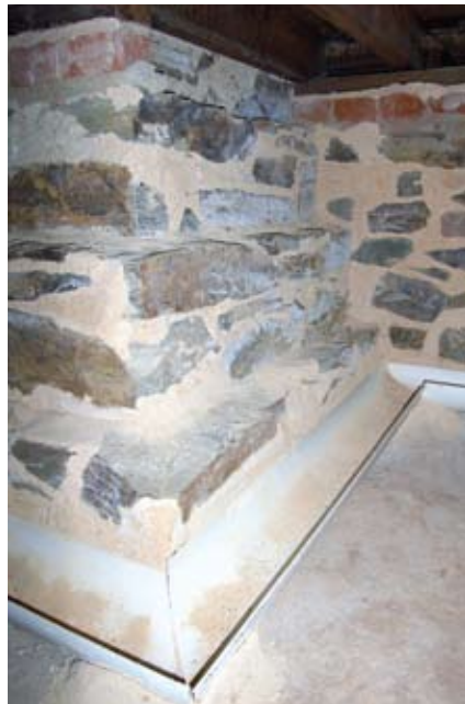
Figure 27 Semi-circular sections of PVC piping catch salt and other debris from sacrificial plasters and mortars on the walls beneath the floor of a church. Bedded on the same sacrificial mortar mix as that used for the walls, the pipes prevent the recirculation of the salts through the soils below and are cleaned out annually. White salts are visible on the stones in the centre of the photograph.
