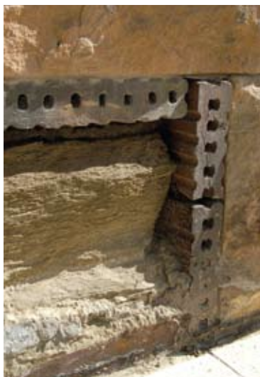
Figures 9 and 10 Hard burnt and glazed ventilating ceramic tiles and bricks. Made for the purpose, these are among the best dampcourses ever used, particularly the example at left from 1879. At right is a 1930s example which (together with its adjacent brickwork) is a remedial undersetting of an 1840s church of rubble limestone. Both examples were laid with open perpendicular joints to prevent damp travelling through the permeable mortar. In both cases salt attack is damaging the masonry below the DPCs — and each building will need treatments to control the salts (see Sections 13 & 14).
