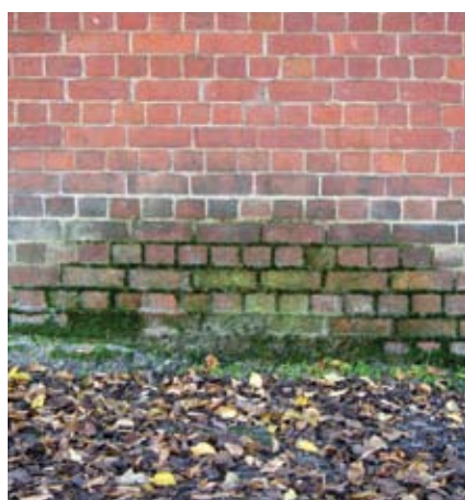
Figure 23 Maintenance, maintenance, maintenance. Here a roof gutter has rusted through and the colourful green damp zone is due to splash.
